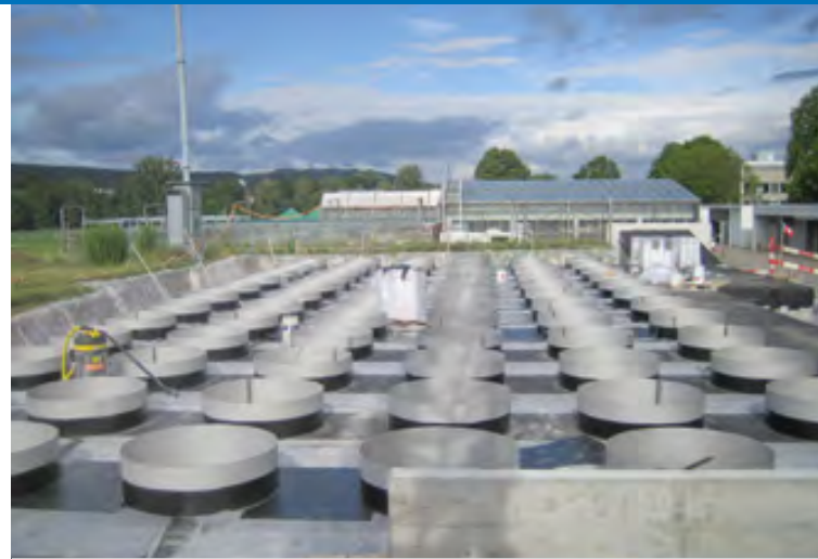
Planning and installation of complete measurement stations
